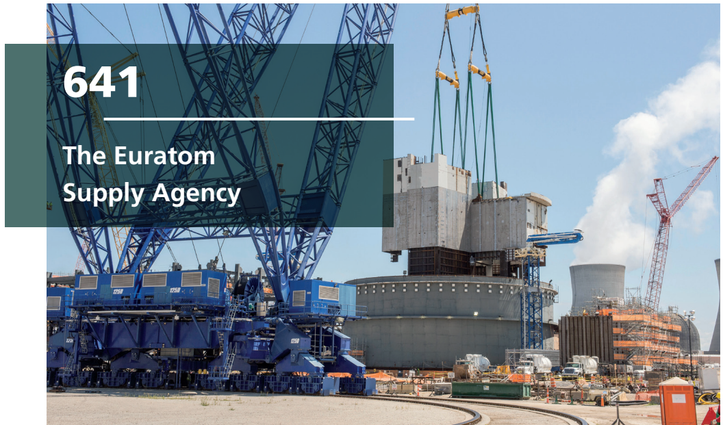
The large heavy lift derrick places the 1,200 ton CA01 module into the nuclear island of Vogtle Unit 3. Two Westinghouse AP1000 nuclear units with approx. 1,117 MW each are currently under construction at the Vogtle site, Burke County, Georgia, in the south-eastern United States. Commissioning is expected for 2019 and 2020, respectively. (Courtesy: Georgia Power Company)
